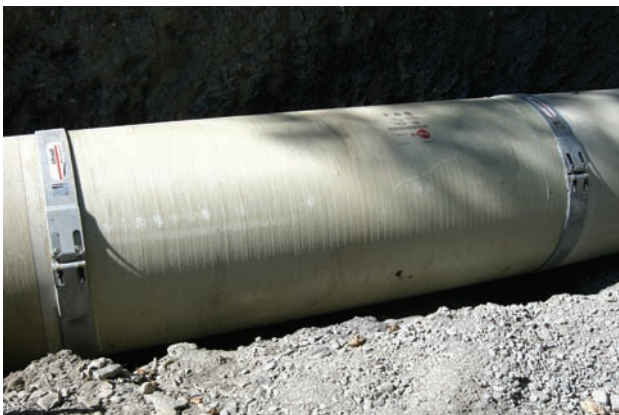
For the installation of an adapter piece
