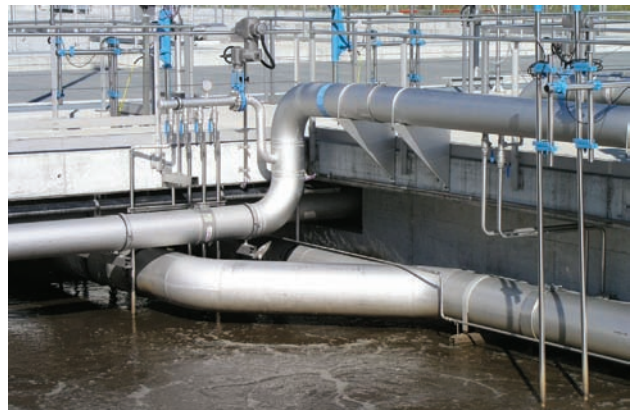
Prefabricated pipe section are installed with STRAUB-GRIP-L
